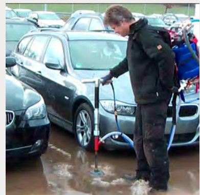
Injected air makes dense subsoil permeable
